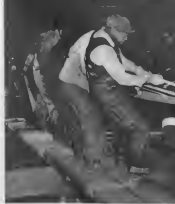
DEEP within the ways, a shipyard crew swings a battering ram to knock the shores from beneath a super tanker. Minutes later a bottle of champagne will be cracked across her bow and . . .
